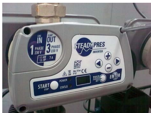
Open the front cover by unscrewing the 4 screws
