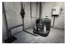
The lifting unit is installed in a space below the backflow level. Sewage from all drainage objects below the backflow level flows into the lifting unit. On the discharge side, the lifting unit is connected to the sewage system above the backflow level via a pipe loop. Inlet and discharge lines are self-supporting.
